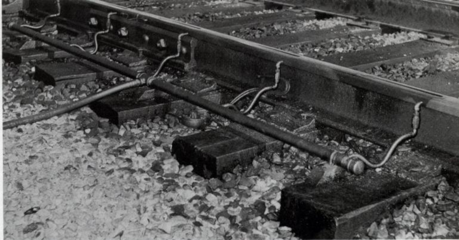
RAIL SURFACE OILERS used just beyond group retarders at Big Four Yard lubricate wheels and rails, permitting cars to roll more uniformly.
