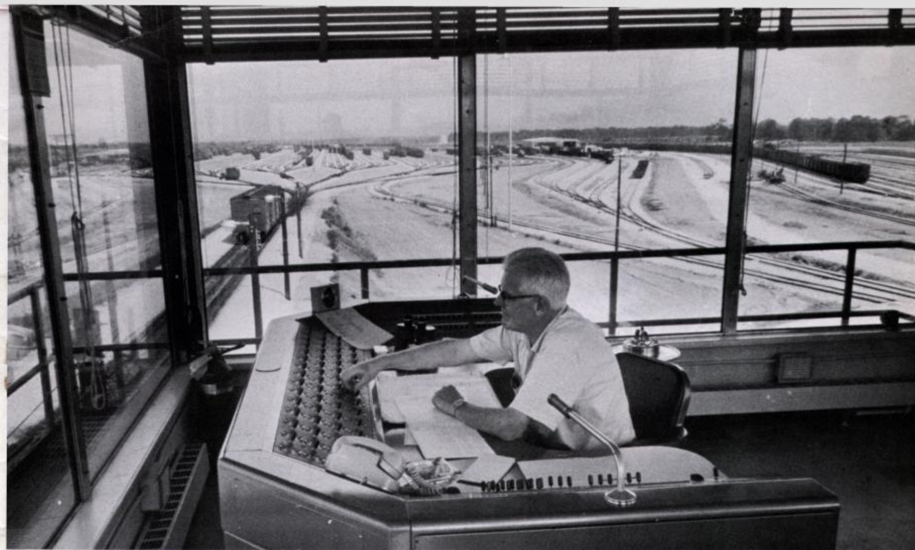
YARDMASTER'S console atop hump tower at Big Four Yard. Panel contains counters that show how many cars are in each classification track.
