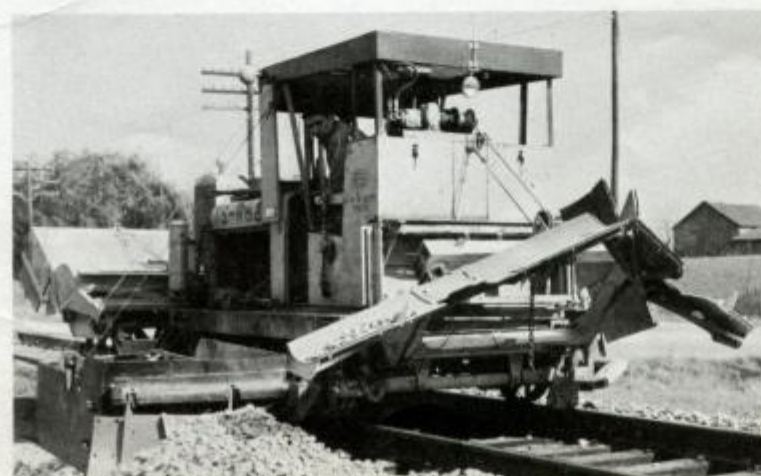
BALLAST REGULATOR is used with NYC's tie and surfacing gangs.
