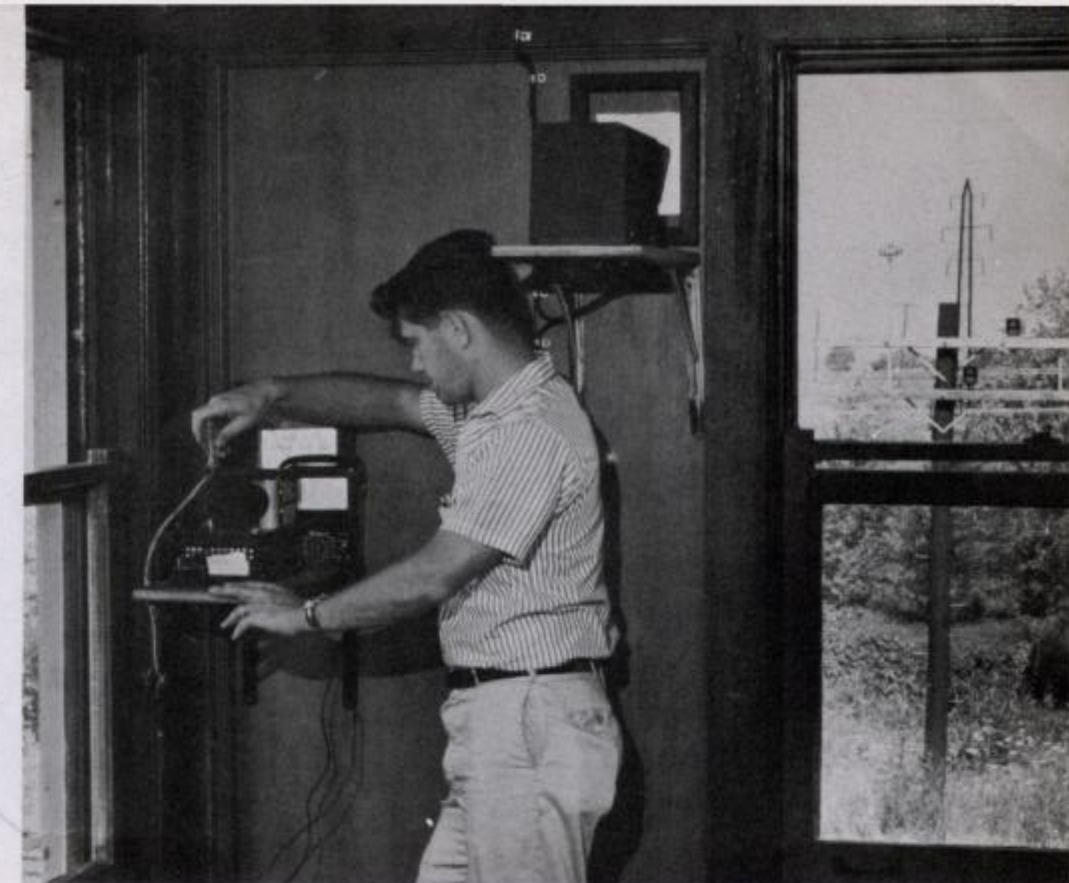
HIGH-LOAD DETECTOR is a recently-developed device. When a passing load is dangerously high, it interrupts a light beam and sounds an alarm.
