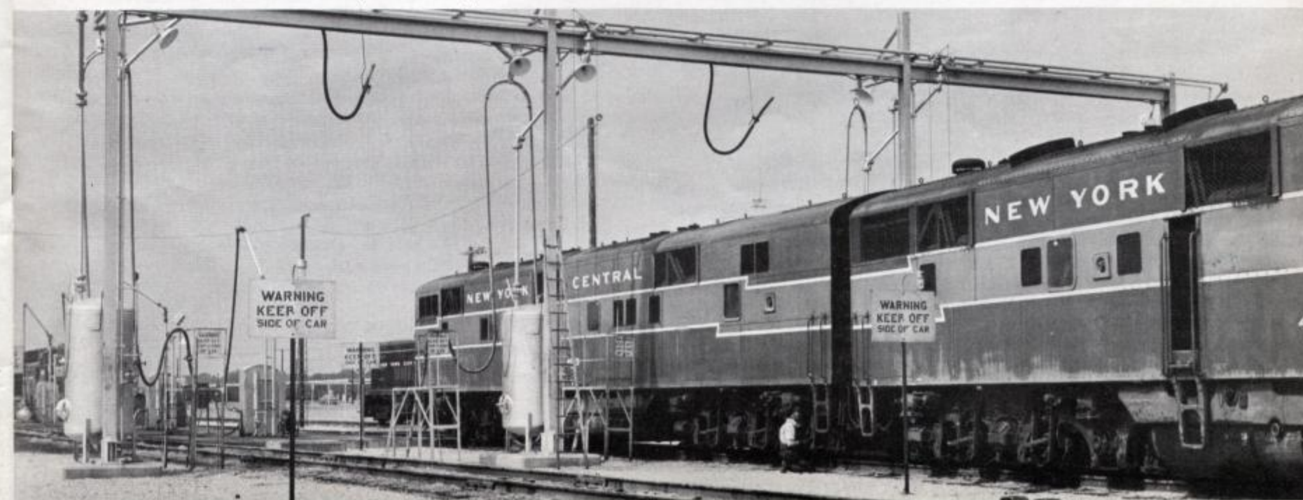
DIESEL SERVICE CENTER at Big Four Yard typifies modern New York Central locomotive facilities. The gantry structure carries sanding hoses.
