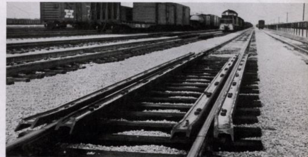
SPRING RETARDERS, installed at Big Four Yard, stop cars when they approach the fouling point. They're more effective than conventional skates.
