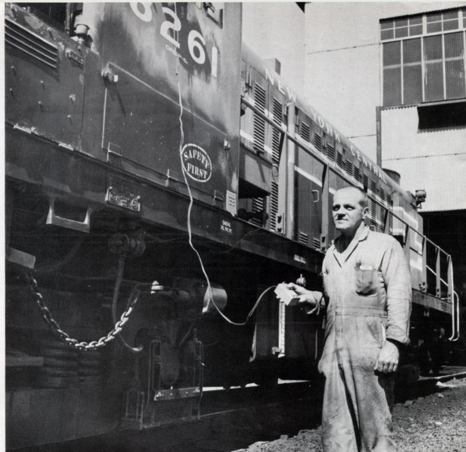
"BUG" moves coupled diesels through spot service shops. Pressing button applies battery power to traction motors.
