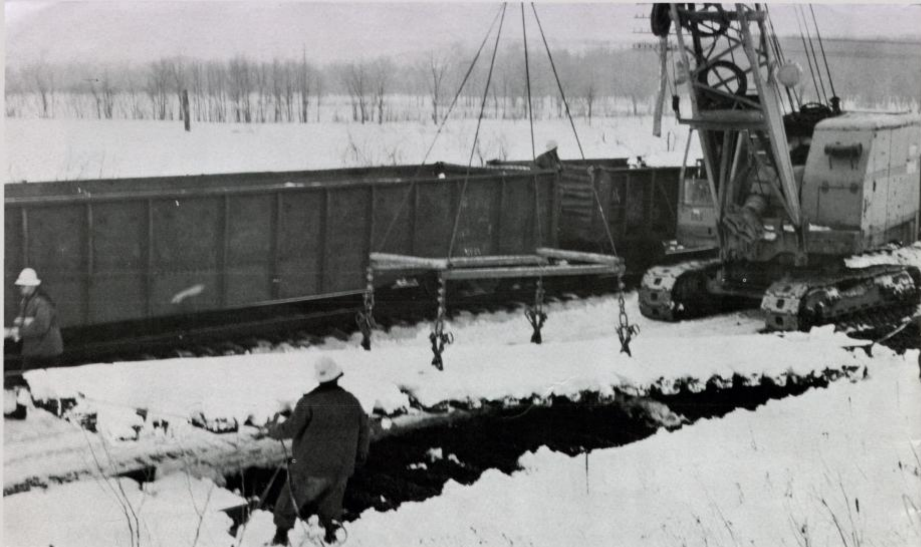
TRACK PANELS, removed from Syracuse division main line when CTC was installed, are loaded on gons for transfer to Indianapolis, to be laid in new electronic yard. Second hand panels cost about a fourth as much to lay as conventional track in yard construction.
