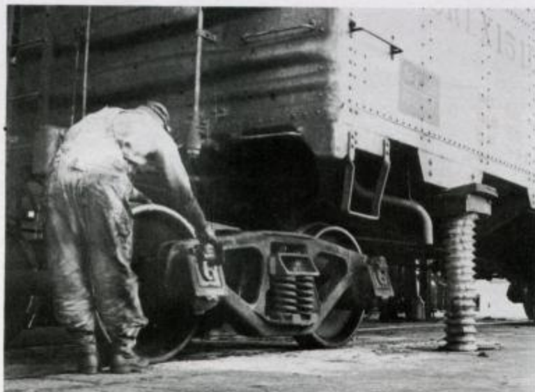
ELECTRIC JACKS raise car ends for removal of trucks at Robert R. Young Yard, Elkhart (shown here) and at Big Four yard. Central uses spot system for both car and locomotive maintenance, finding it greatly increases efficiency and cuts out-of-service time for equipment.
