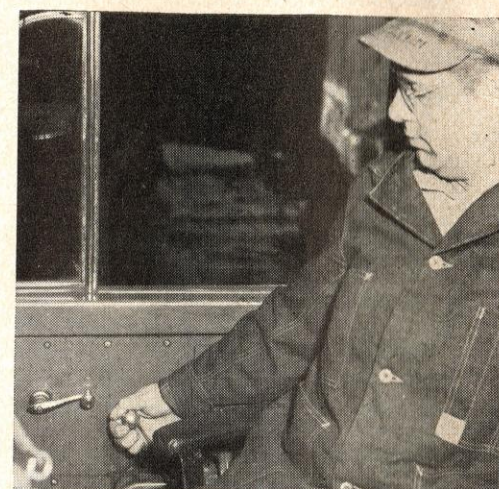
TO LET INDUCTOR "know" he has observed signal, engineman* operates fore-staller. If he didn't, train would stop.
