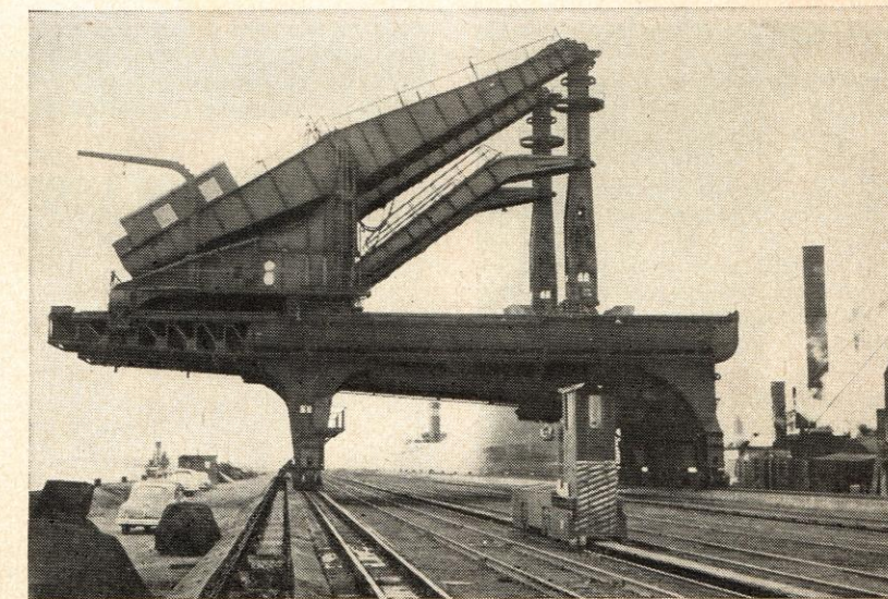
THIS PAIR of ore unloaders at Toledo, O., docks will be remodeled; two new 20-ton ones are to be installed (see story, opposite page).
